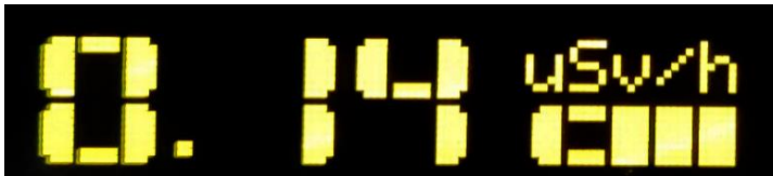
Figure 27– DER value during backup power supply
